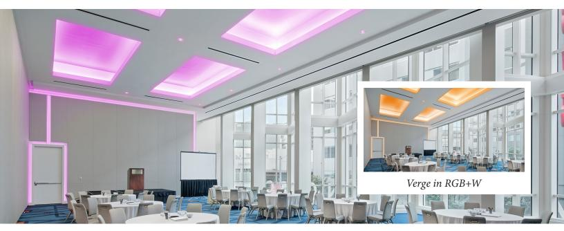
The Verge lighting system was installed on the door frame, and into the corner of where two walls meet while also going horizontally along the top of the wall where the wall meets the ceiling, as well as the vertical line above the doorframe. The design team chose Verge in RGB+W to feature changeable accent colors to portray event/company branding.
